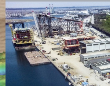
First Steel Cut at Rosetti's Ravenna yard
