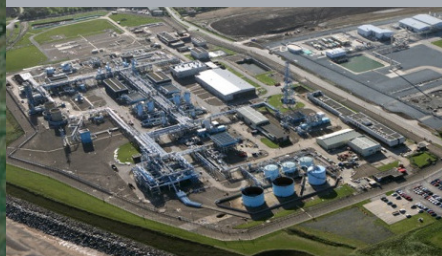
Centrica's Easington Terminal
