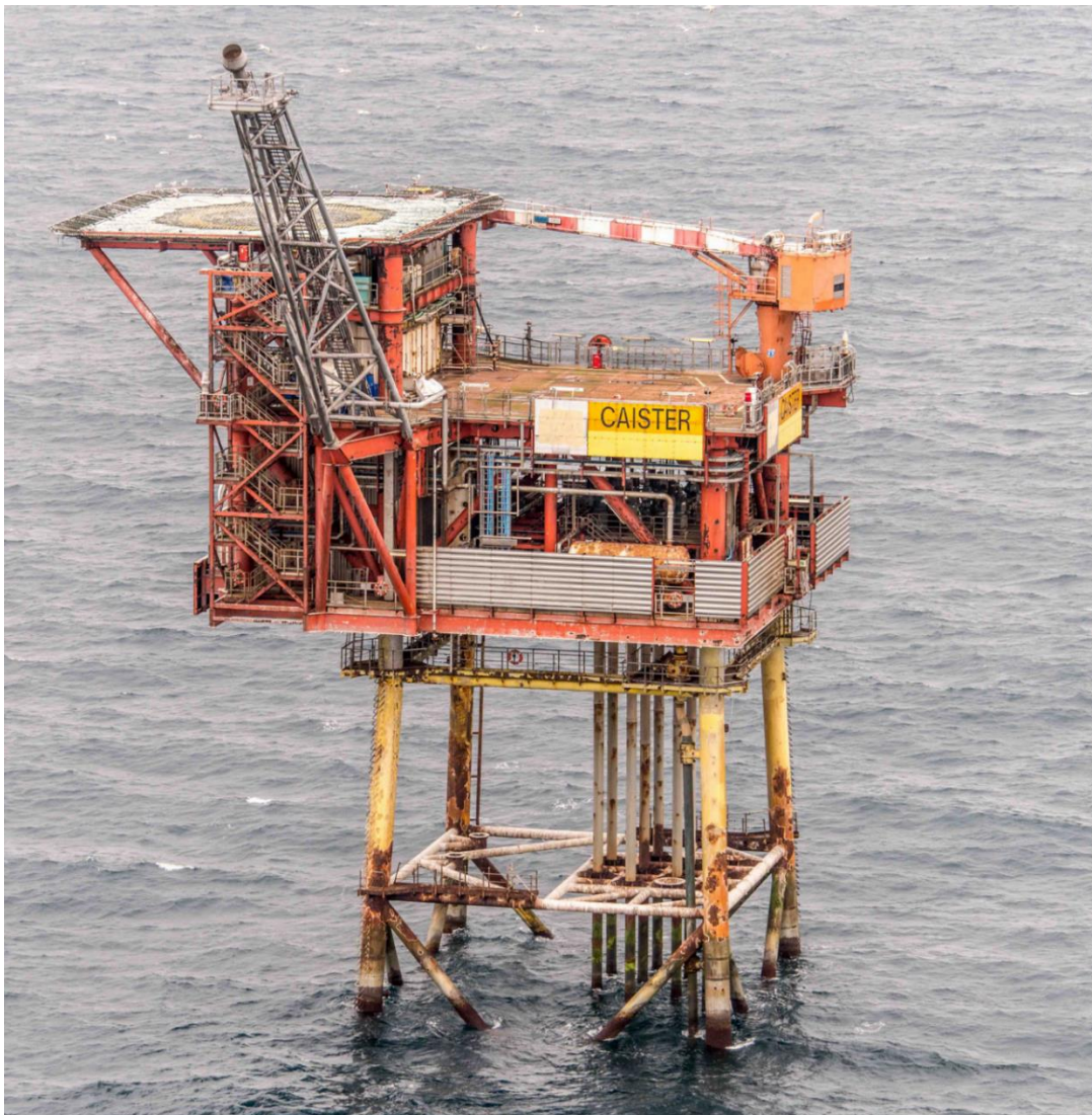
Figure 2.1.1 Photograph of Caister CM Platform
