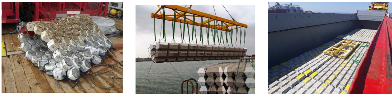
Figure 2.4.7: Linklok, Fleximat and Biflex mattresses respectively (indicative only)
