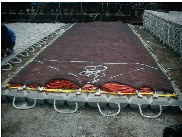
Figure 2.4.3: Typical Froned Mattress Types (gravity based & anchored) 10
