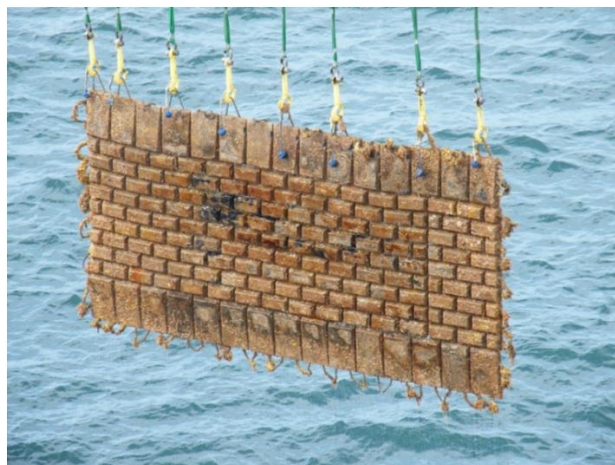
Figure 5.4.1: Removal of a mattress using a 'curtain' lift
