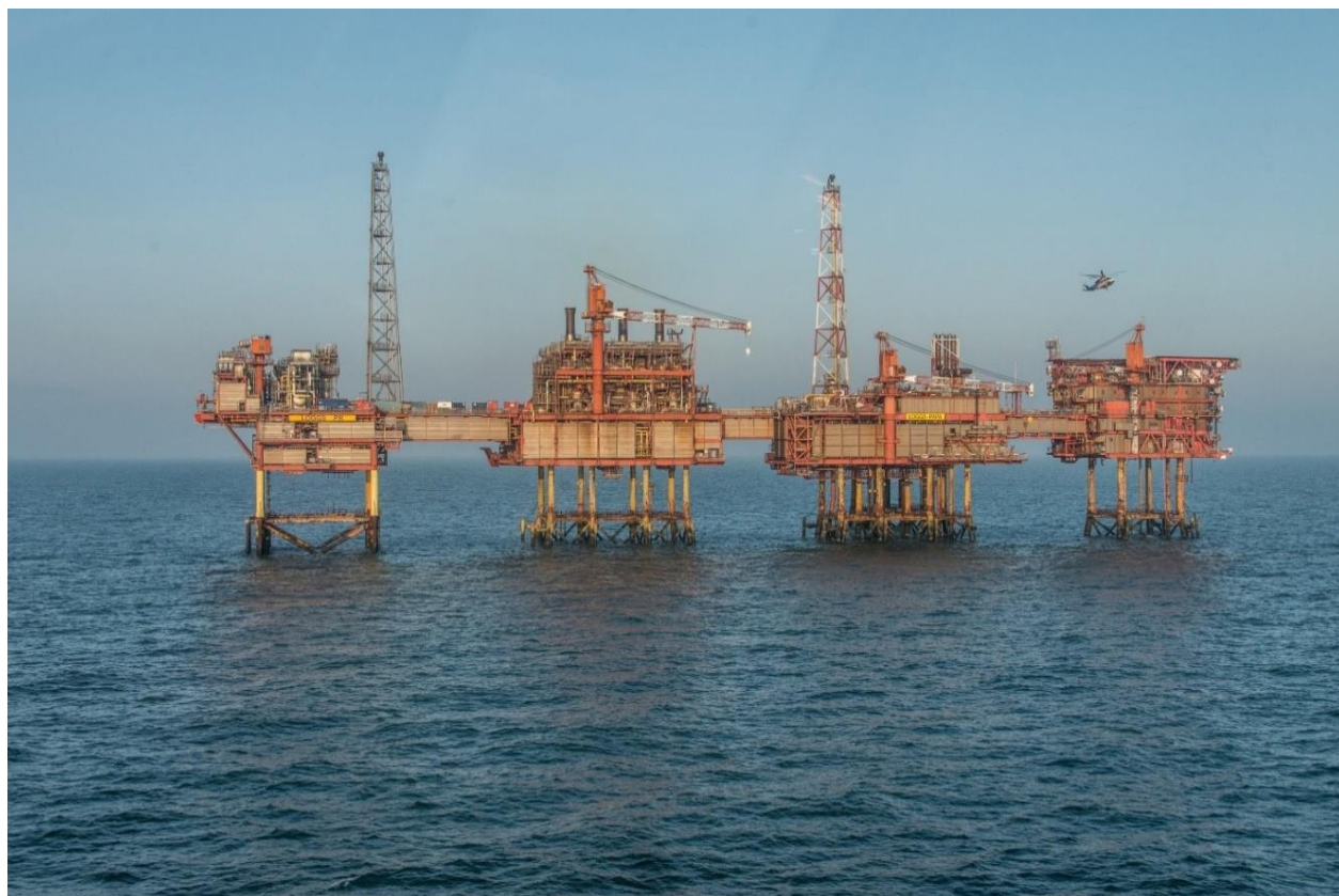
Figure 2.1.3: Photograph of the LOGGS Installation, View Looking North
